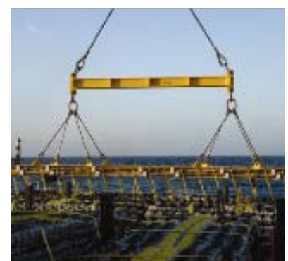
Mattress Installation Support
