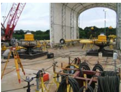
Fabrication Yard Survey
