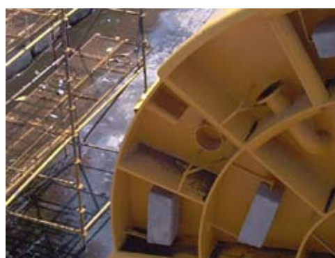
Pile Installation Survey
